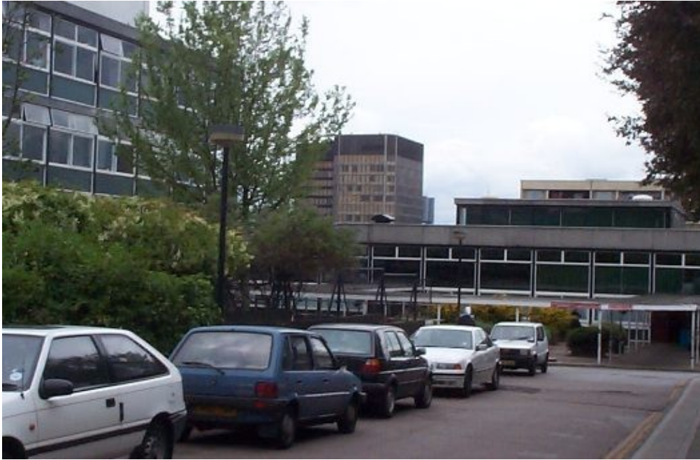
Elizabeth Garrett Anderson School, Islington – an inner urban school.
