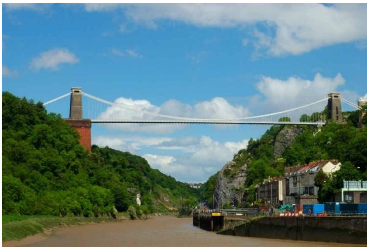
The Clifton Suspension Bridge in Bristol
