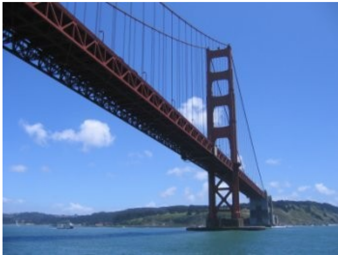
The Golden Gate Bridge in California
