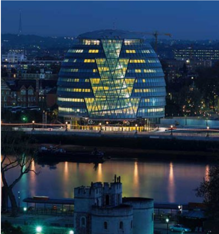
The London City Hall on the river Thames. Note the giant helical stair case inside. Image © Foster + Partners.
